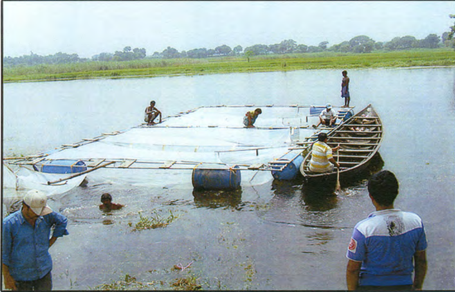
Cage fabrication and installation at Kalindi Wetland
