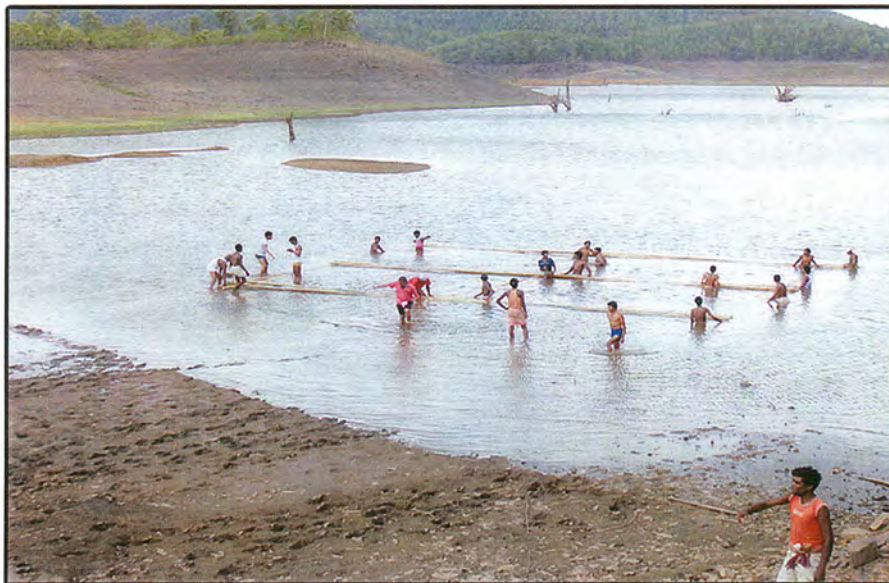
Cage Construction in a Reservoir
